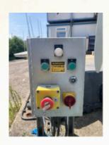
Unlock emergency stop button and turn isolator to "ON" Carefully lay out winch rope and attached pulley to the strong point.
